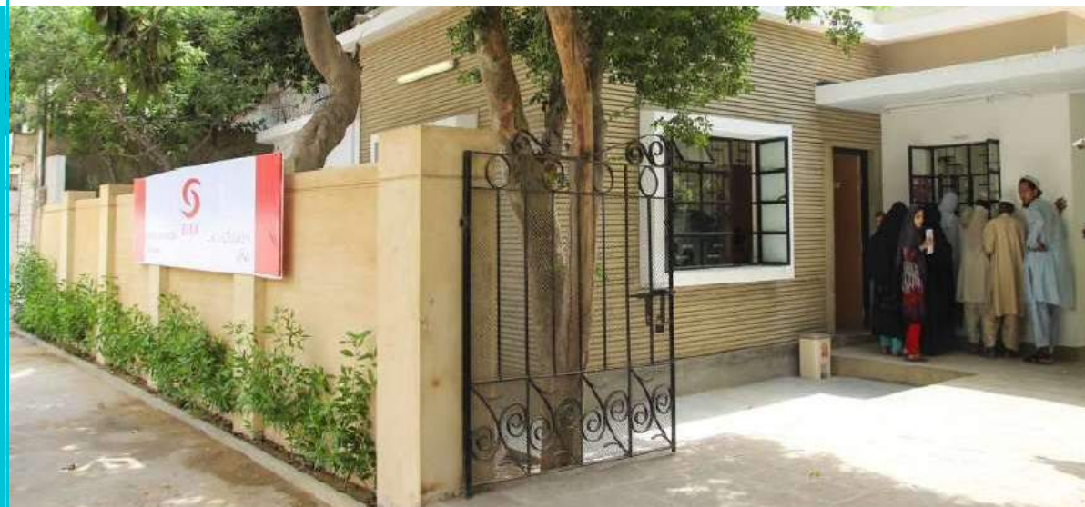
Exterior after renovation process
