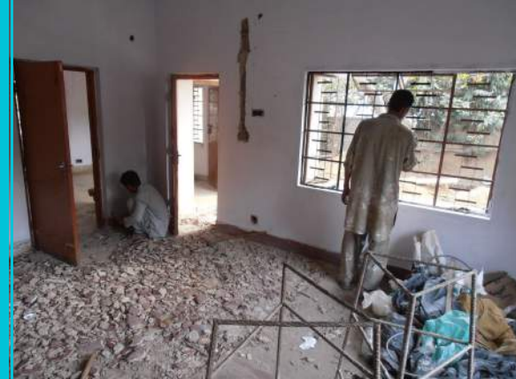
Interior of the clinic during the renovation
