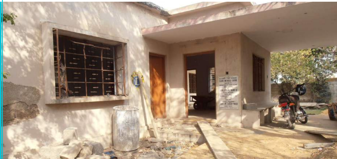
Exterior in process of renovation
