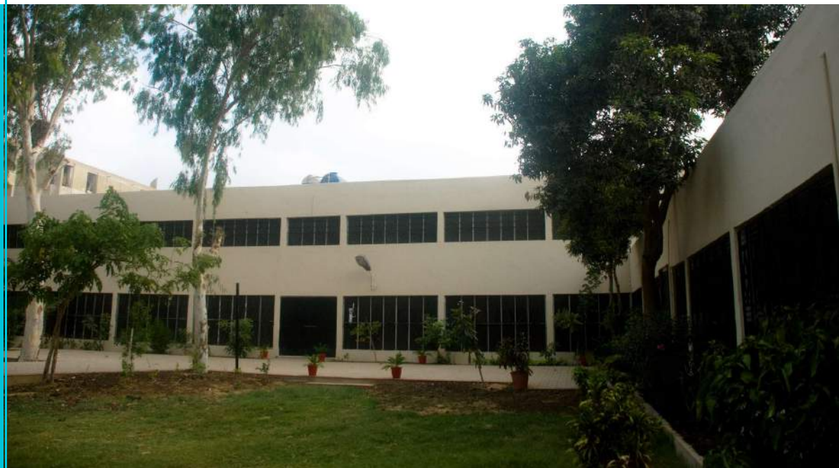
Facility of Panah Shelter Homes located in FB Area, Karachi
