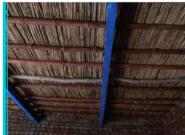
The roof structure
